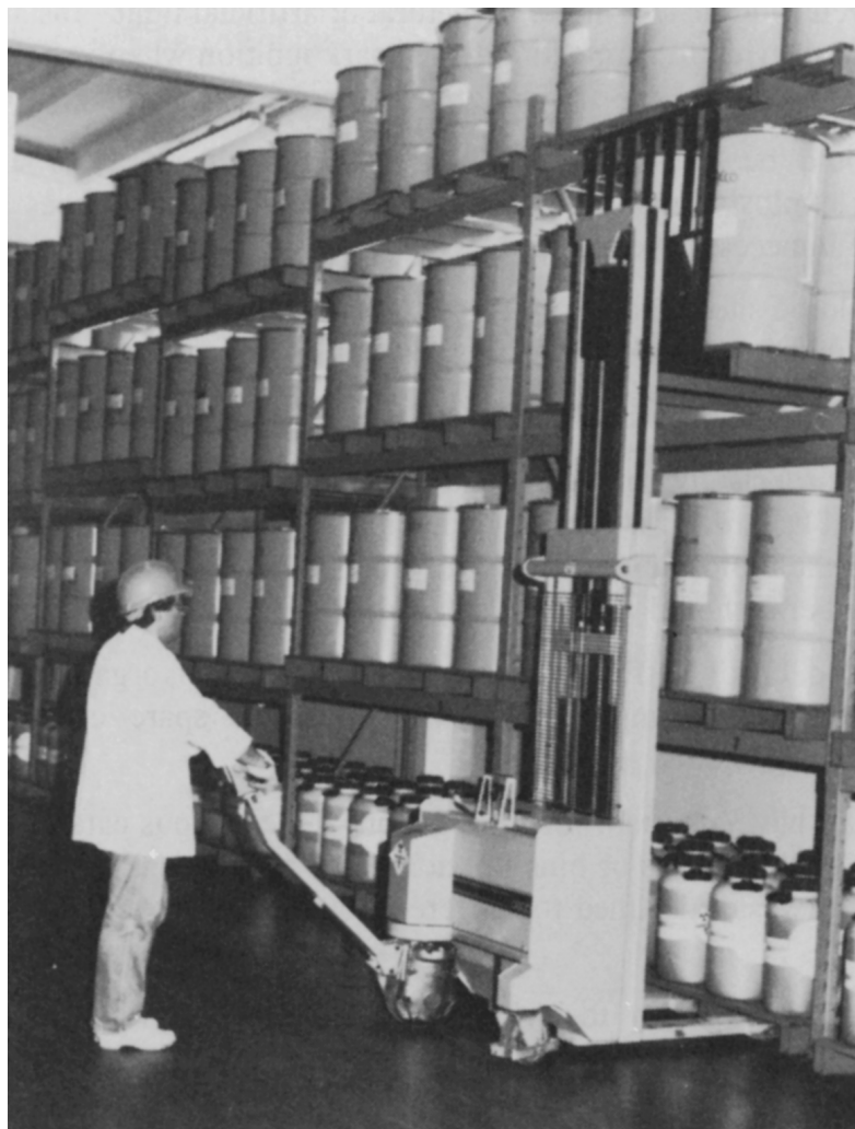
FIG. 4. View of the decay storage facility during loading of radioactive waste.
